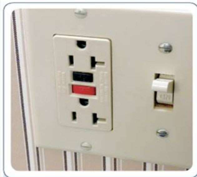
EXHIBIT 210.8 A 15-ampere duplex receptacle with integral GFCI that also protects downstream loads.
