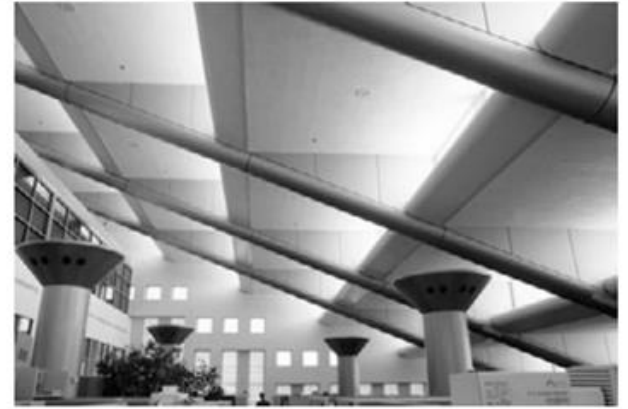
PHOTO 20.39 Stepped windows and light shelves throw natural light deep into the building. (Courtesy of NREL/DOE)
