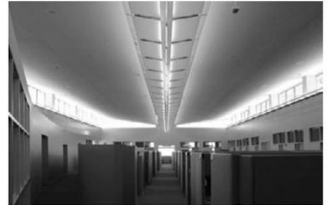
PHOTO 20.40 Side lights and a roof monitor in the center of the ceiling throws natural light evenly. (Courtesy of NREL/DOE)
