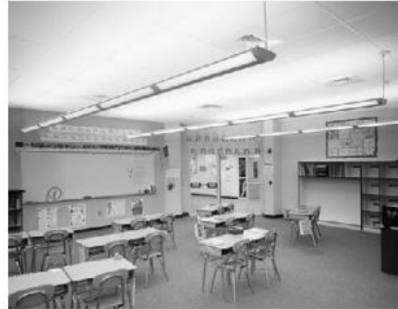
PHOTO 20.26 A classroom space lit with uplights, a more comfortable seeing environment because there is less glare. (Courtesy of NREL/DOE)
