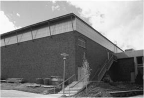
PHOTO 20.35 Exterior windows designed to introduce daylight in a gymnasium. (Used with permission of ABC)
