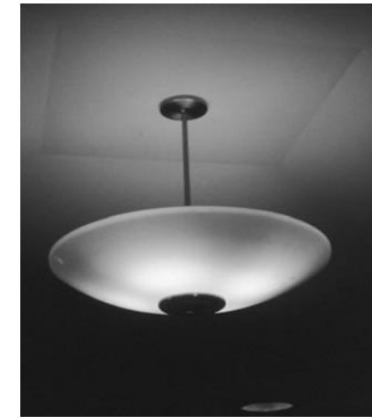
PHOTO 20.8 A decorative pendent light suspended from a ceiling, which provides ambient lighting. (Used with permission of ABC)
