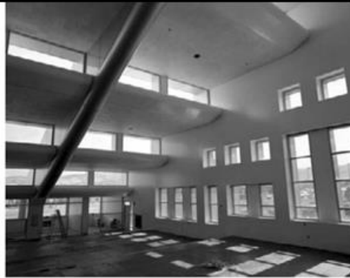
PHOTO 20.38 Stepped windows provide soft, natural lighting to the open office area below. (Courtesy of NREL/DOE)
